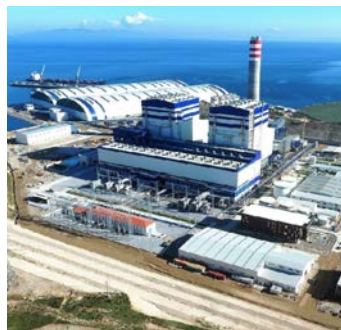
CENAL Power Plant, TURKEY
