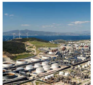
Star Refinery, TURKEY
