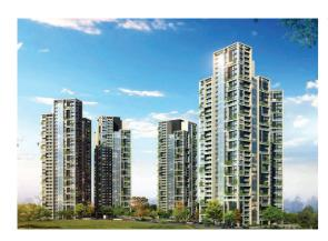
The project consisting of 6 buildings with a total of 770 apartments. In the project with a total of 36.000 sqm insulating glass, Sisecam Temperable Solar Low-e Neutral 62/44 is being used.
