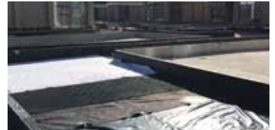
Roof Drainage and Insulation
