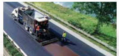
Asphalt Protection System
