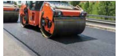
Recycling of Asphalt
