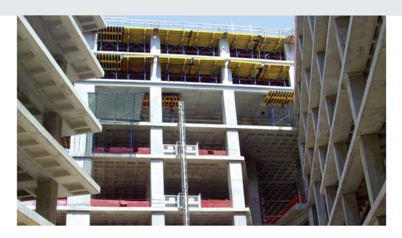
The major part of slabs was statically sorted out with "coffered slab". HD 150 slab table system is very useful in these types of slabs with a few beams. Tables are covered wholly with plywood. This method which was a little expensive as initial investment reaped a huge profit by the end of the project by developing both productivity and labour safety.
