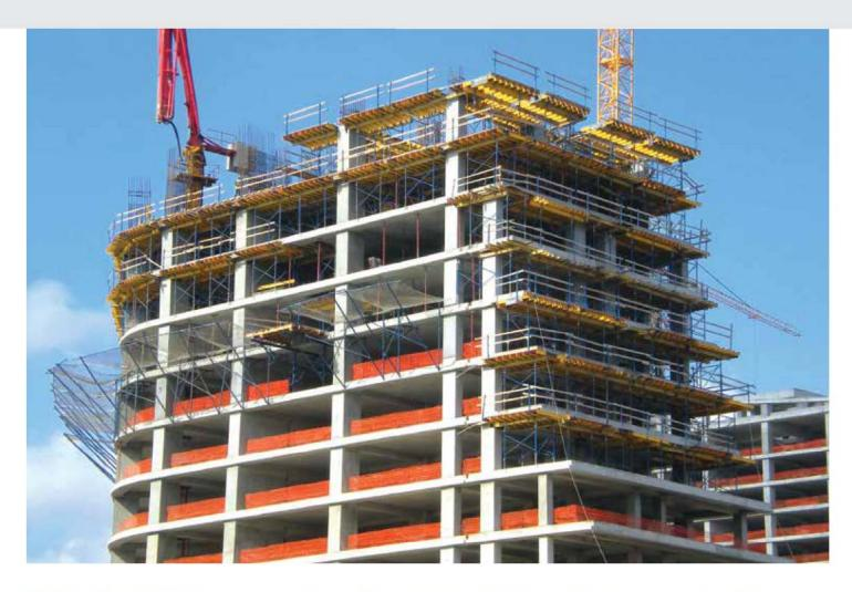
"HD 150 Tableform System" was used on slab formwork. If a project is appropriate as a form, there are a large number of floors identically repeating the same and tower crane has enough time, tableform system is a distinguishing solution. This system provides not only enormous labour productivity but also tremendous economical benefit by preventing damage of formwork material.
