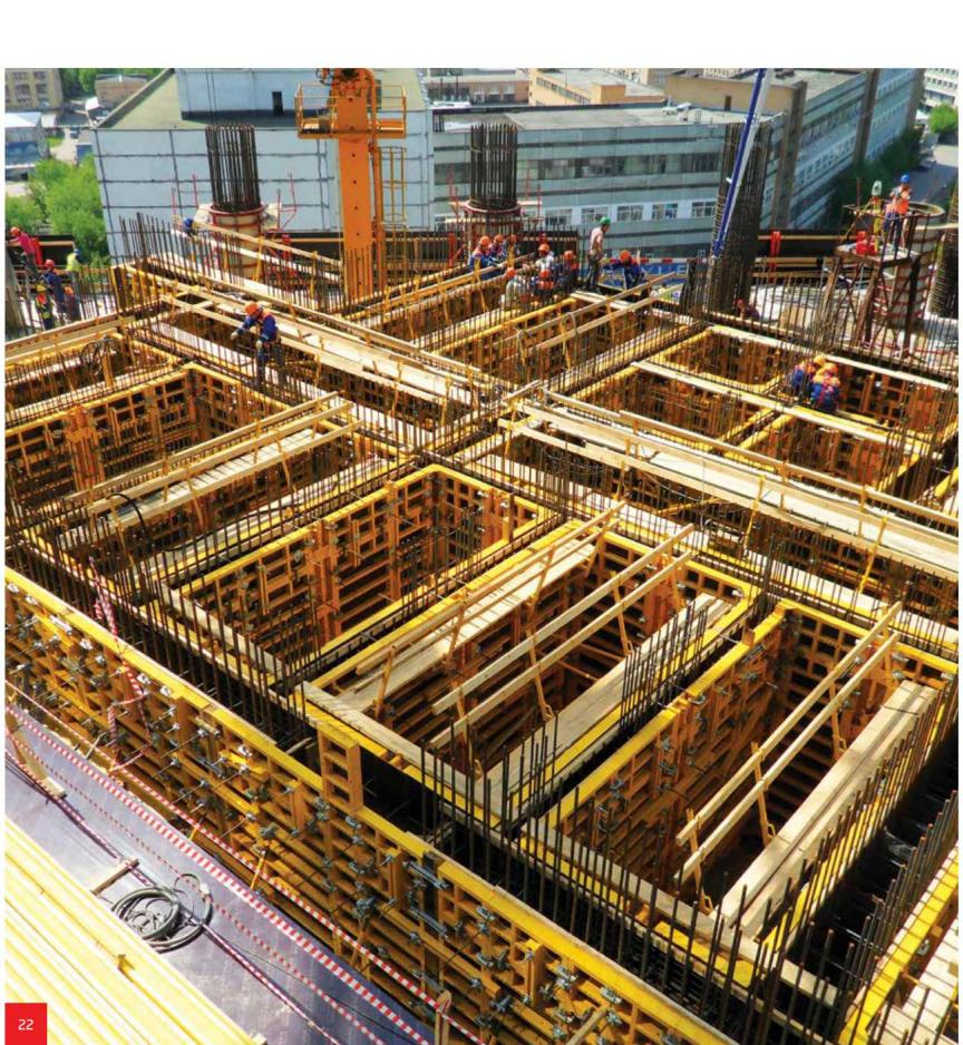
At 47-storey A block, special application of PANEMAX system, "reducable shaft wall formwork", was used in core wall at type floors in a size of - 1.800 m². The formwork installation time at core walls with an area of -1.200 m² in height of 360 cm reduced up to 4 days.
