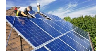
Roof Application Installation
