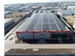
Roof Ges Projecting and Installation
