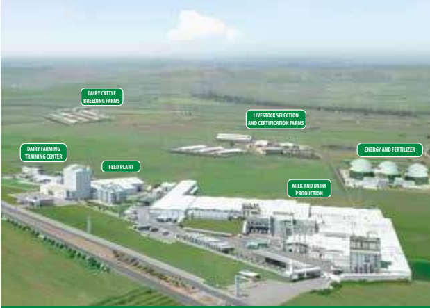
SÜTAŞ KARACABEY INTEGRATED FACILITIES
