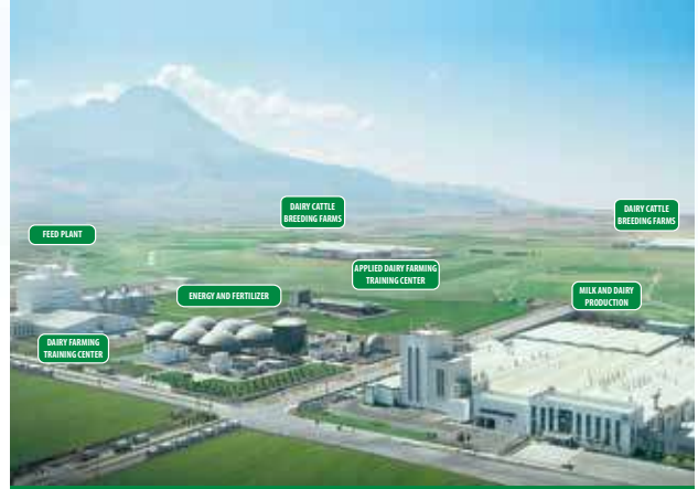
SÜTAŞ AKSARAY INTEGRATED FACILITIES
