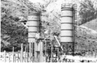
Beton Santrali Conc. Batching Plant
