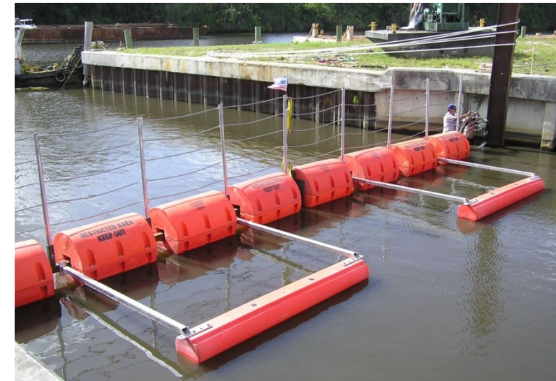
WATER SUPPLY DAMS
