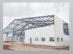
We supply insulated 3 ribs and 5 ribs Rigid polyurethane (PUR) and polyisocyanurate (PIR) sandwich panels. The high thermal properties of sandwich panels make them suitable for insulated roofs, cold rooms, roofing, wall partitioning and insulated sheds. They are also appropriate for containers, portable cabins, prefabricated houses, and shelters.
