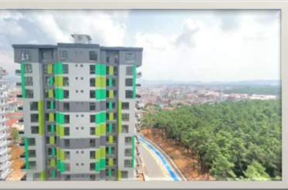
Turan İnşaat Golden Park (Taşdelen) 132 Apartment
