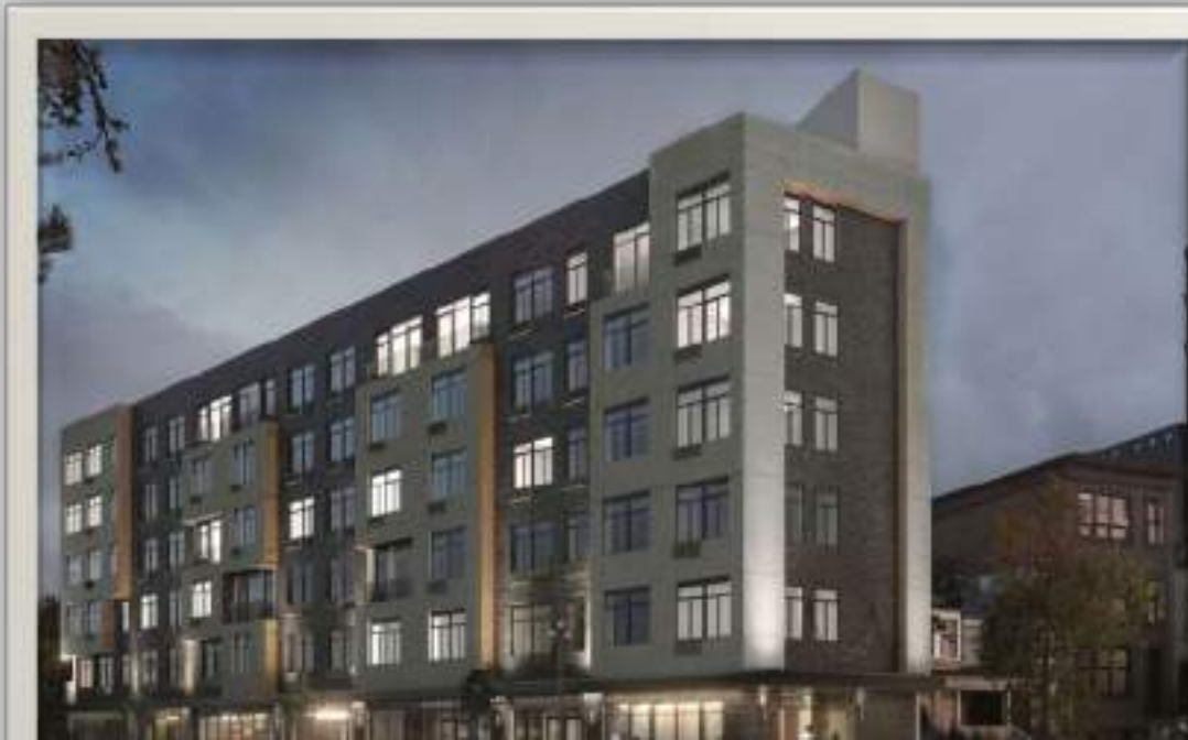
RIG Construction 99 Storms Ave (New Jersey) 50 Apartment
