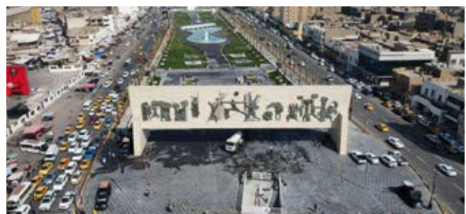
TAHRIR SQUARE, MANUMENT RENOVATION BAGHDAD / IRAQ
