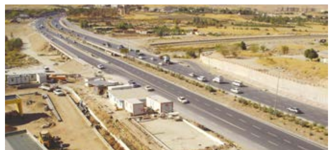
SULAYMANIYAH BRIDGES AND ROAD SULAYMANIYAH / N.IRAQ
