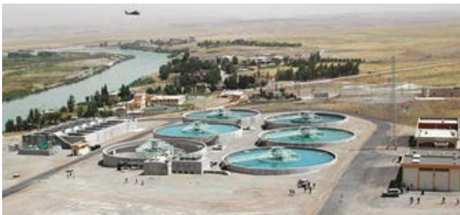
IFFRAZ WATER TREATMENT PLANT ERBIL - N. IRAQ
