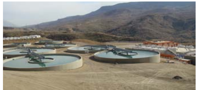
DOKAN WATER TREATMENT PLANT DOKAN - SULAYMANIYAH / N.IRAQ
