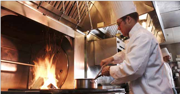
Restaurant Fire Suppression System
