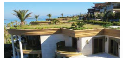
GeoGreen Green Roof
