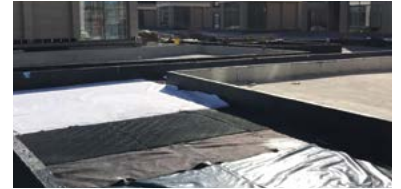
Roof Drainage and Insulation Systems
