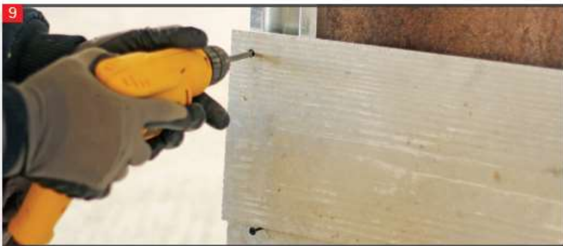
Carbon coated anti rust drywall screws should be used and driven in vertically.
