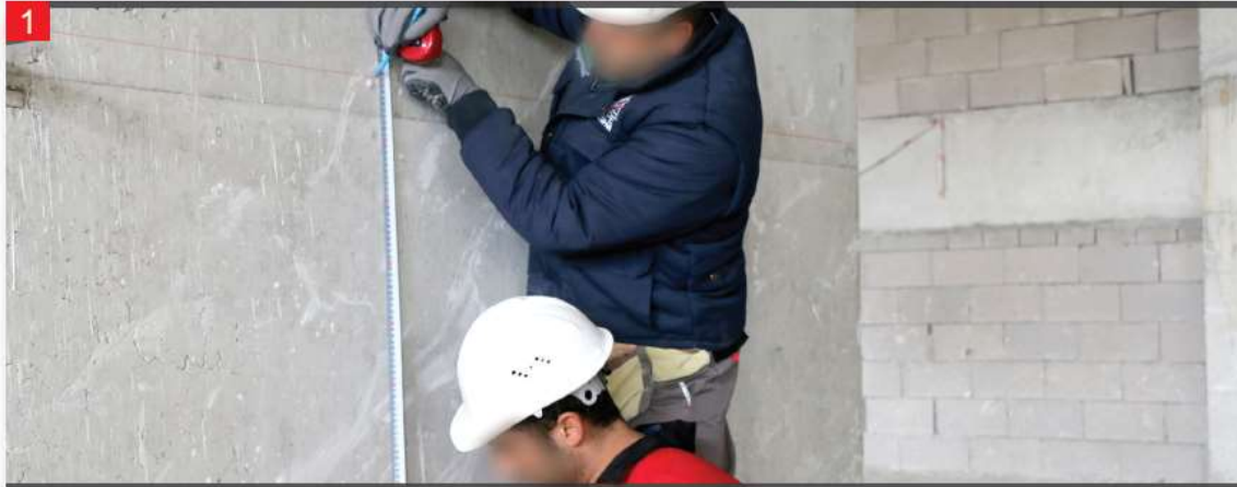
The suitable size of L consoles is selected to level the surface of application and use the desired thickness of insulation material.
