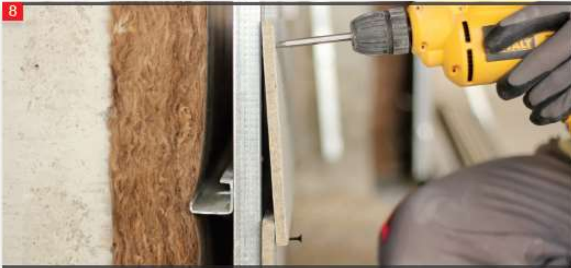
The subsequent overlapping panels are aligned and screwed on the M profile surface
