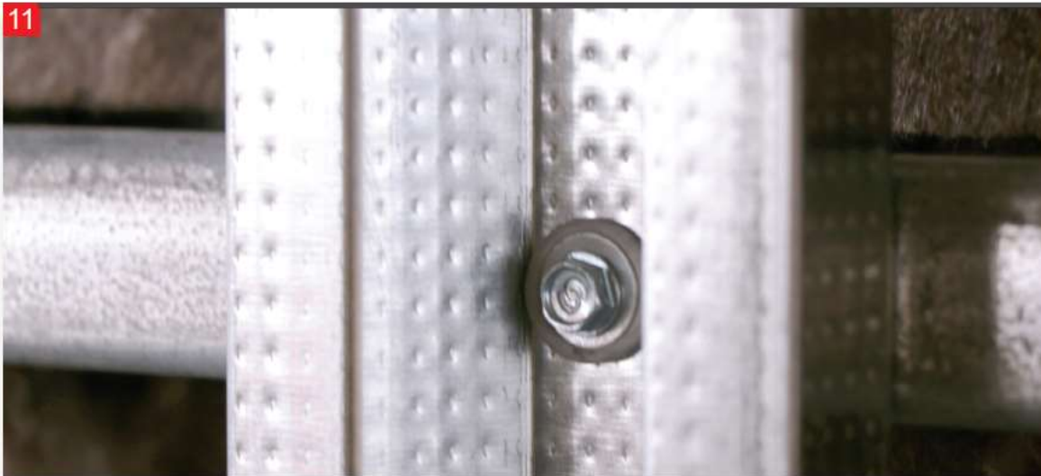
The M profiles are attached to the surfaces of L profiles, for which the leveling has been checked, using triphone self tapping screws screwed on to the center of the L profiles as shown in the photograph.
