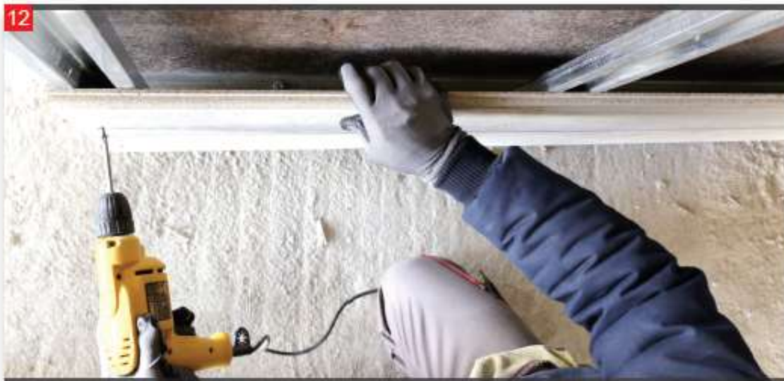
The aligned panels are screwed onto the M profile with anti rust screws.
