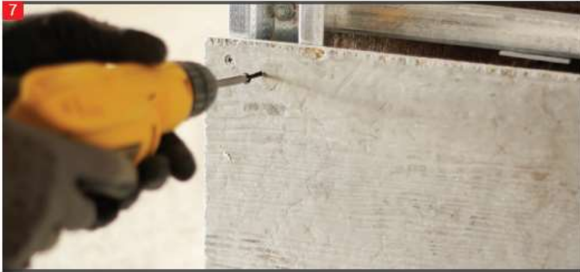
Screws are driven into the measured points as a guide to the overlap panel.
