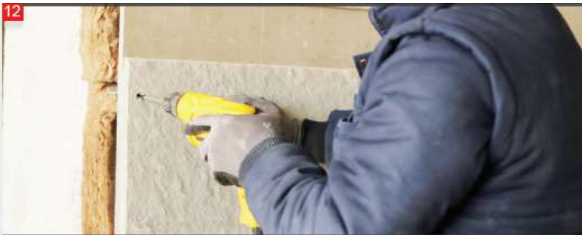
After fixing the laths the next panel is brought over the strips and fixed in.
