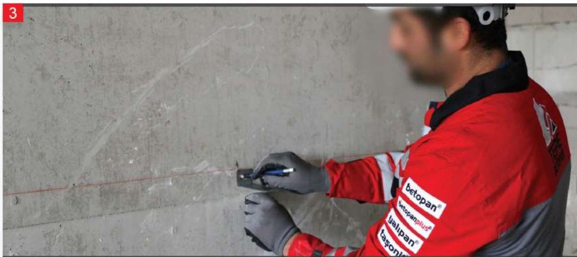
The places to drill for fixing the L consoles to the wall with dowels are marked.
