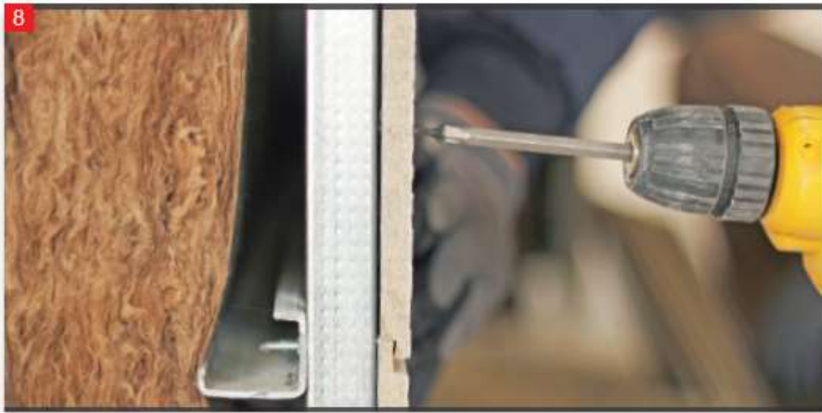
The screws are applied for each M profile and steps 5 through 8 are repeated for all the panels.
