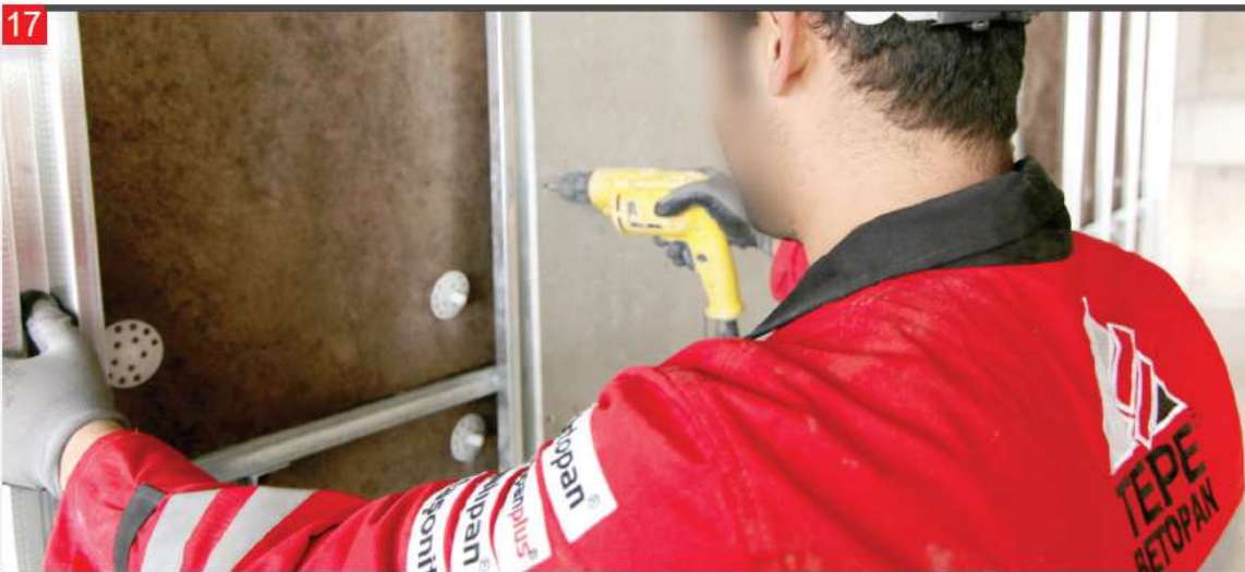
The panels should be screwed onto the M profile wings and during the process of screwing them in, 0.5 mm gaps should be left between the panels to be fixed onto the two wings.
