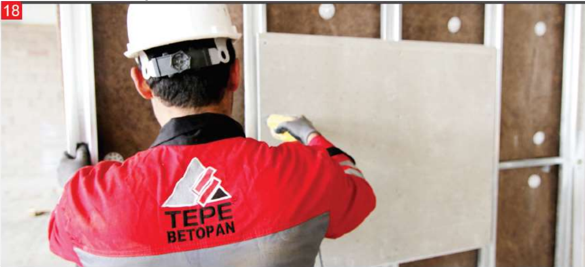
While screwing on the lower and upper sections of the panels 2.5 cm of slack should be left from the upper and lower border.
