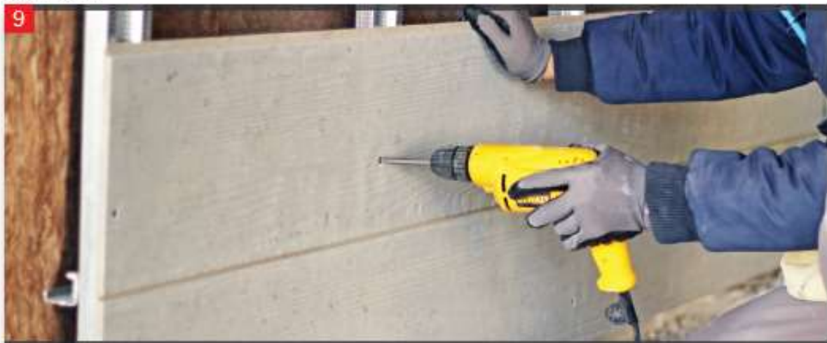
The screws are applied for each M profile and steps 5 through 8 are repeated for all the panels.
