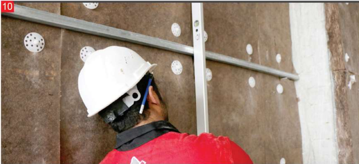
The levelness of the L profiles should be checked throughout the mounting surface.
