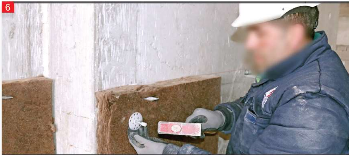
The applied insulation material is fixed to the application surface using parachute dowels.
