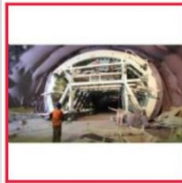
HISARUSTU METRO PROJECT ISTANBUL
