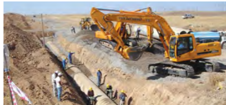
IFRAZ WTP PIPELINE ERBIL / N.IRAQ
