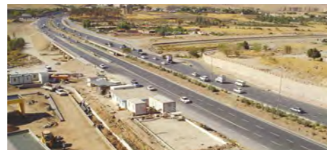
SULAYMANIYAH BRIDGES AND ROAD SULAYMANIYAH / N.IRAQ
