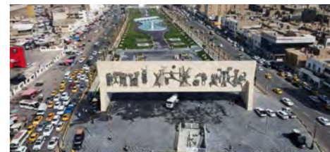
TAHRIR SQUARE, MANUMENT RENOVATION BAGHDAD / IRAQ
