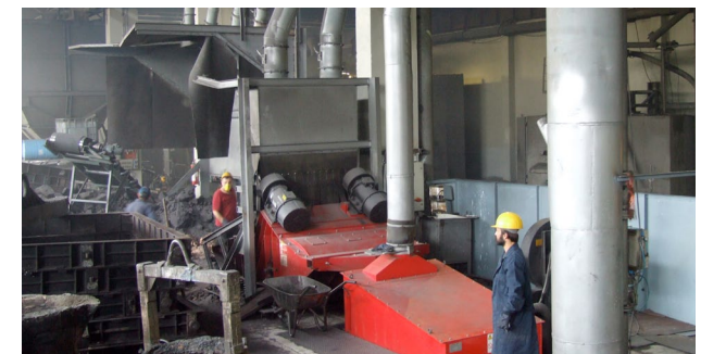
A View From Sand/Reclamation Unit
