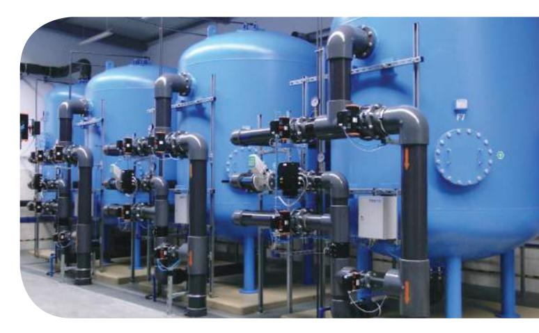
The removal of iron and manganese depends on the type and concentration of the water, which helps determine the best procedure and treatment system. Iron and manganese can be found in water in one of three basic forms: dissolved, particulate, and colloidal. The dominance of one form over another depends on the pH of the water. The two most common treatment methods are removal through oxidation/filtration and adsorption onto ion exchange resins.
