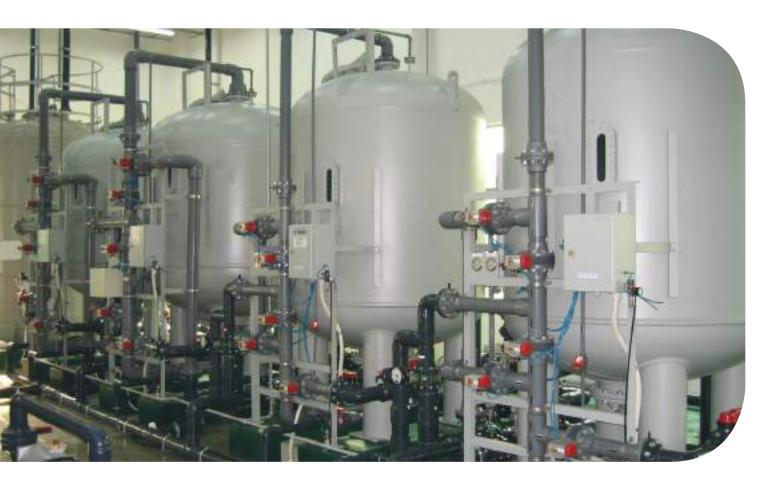
These filters are typically used to remove suspended solids that cause turbidity in water. Their operation is very simple, allowing water to pass through several layers of quartz (sand) and possibly a layer of anthracite. As the water moves downward through the filter media, the materials retained on the first layer of sand enhance filtration efficiency in the subsequent layers.
