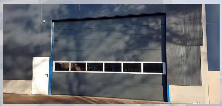
Sectional garage doors, positioned beneath the ceiling, optimize space by opening vertically. This design guarantees maximum space utilization inside and in front of the garage. They can be fitted on any garage opening, offering up to 14 cm of extra clearance compared to solid doors. Moreover, they feature robust insulation with resilient, weather-resistant seals on all sides.
