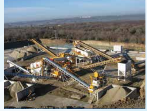
Maden Tesisleri (Mining Facilities)
