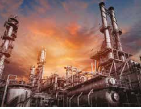
Akaryakıt, Gaz ve Petrokimya Tesisleri, (Oil, Gas and Petrochemical Plants)
