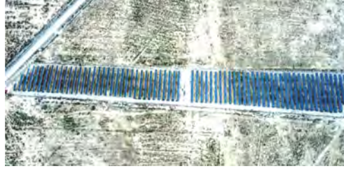
FİNA ENERJİ / 1,2MWp / DENİZLİ / 2018
