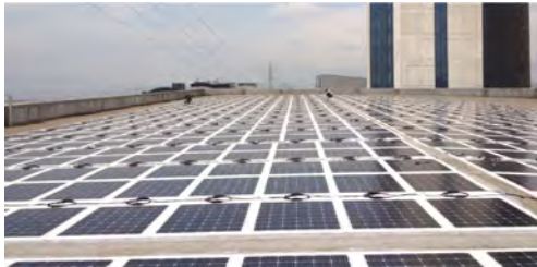
NUH PANEL/ 200kWp / GEBZE / 2016
