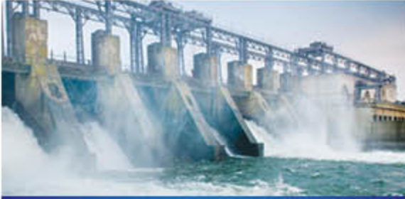
Hidro-Elektrik Enerji Santralleri Hydro-Electrical Power Plants
