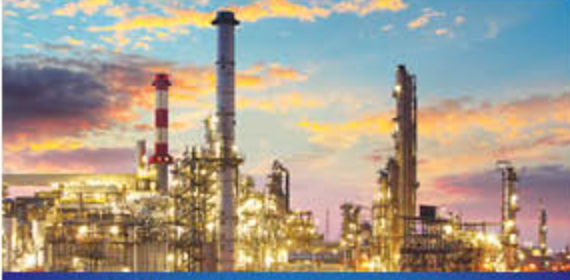
Rafineriler - Petrokimya Refineries - Petrochemical
